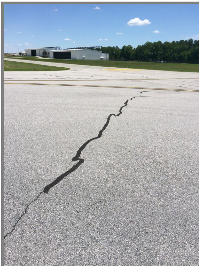
Longitudinal/Transverse Cracking – Taxiway E/F
