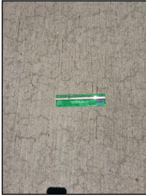
Shrinkage Crack
