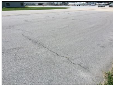
L&T Crack
