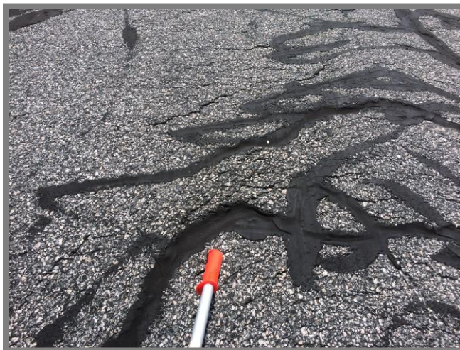
Slippage Cracking – Taxiway G
