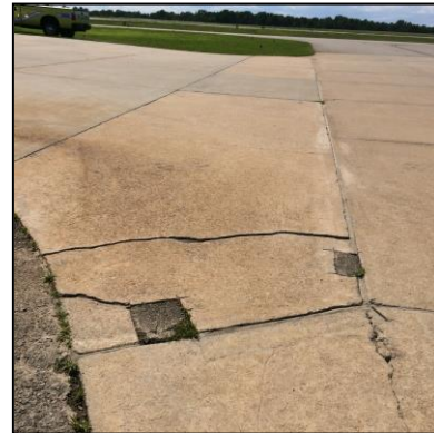
Corner Break, Corner Spall and Small Patch
