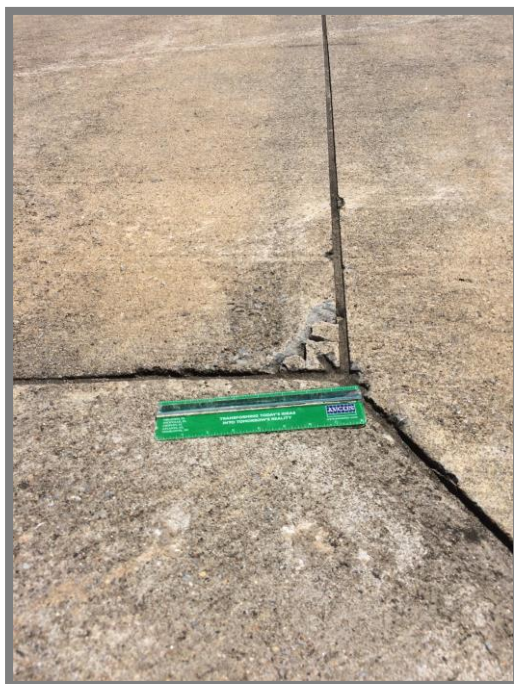
Corner Spalling – Taxiway L9
