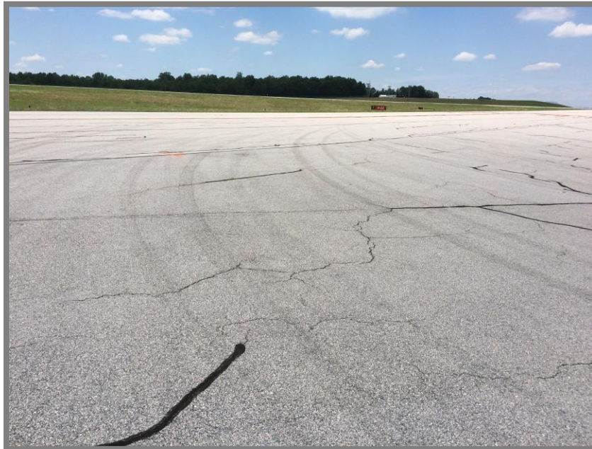
Block Cracking – Taxiway F & Taxiway L Intersection
