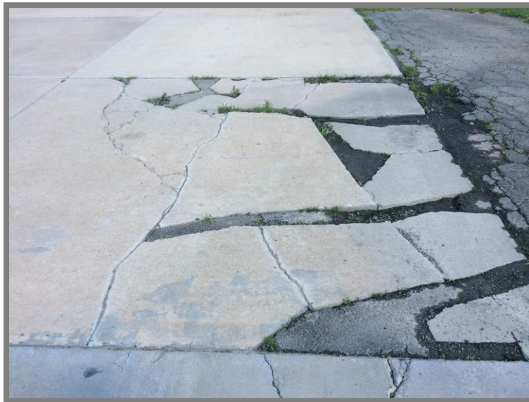
Shattered Slab – Fire Station Apron
