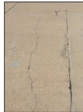
Linear Crack, Joint Spall and Corner Spall
