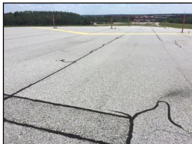
L&T Crack
