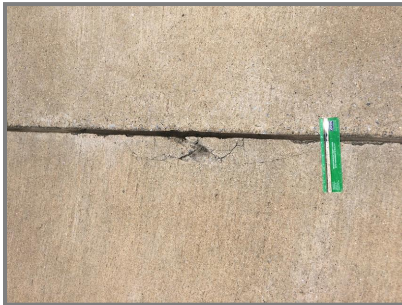
Joint Spalling – North Cargo Area
