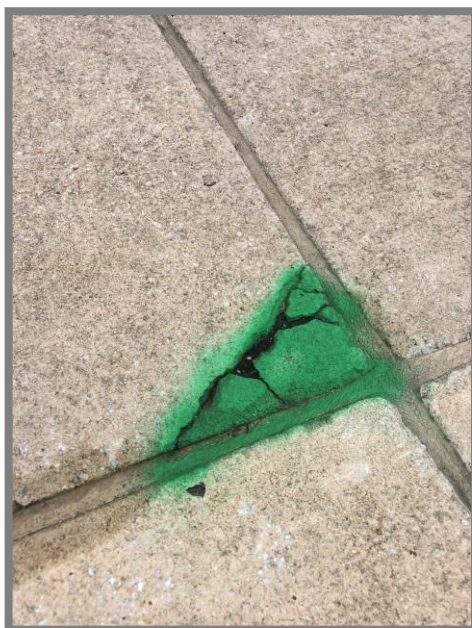
Corner Spalling – Hangar 1
