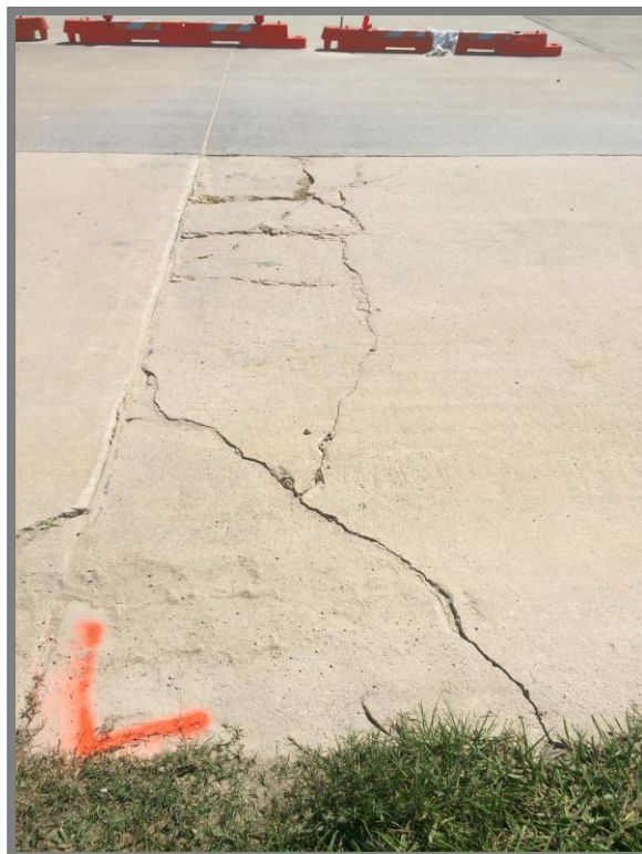
Shattered Slab – Fire Station Apron
