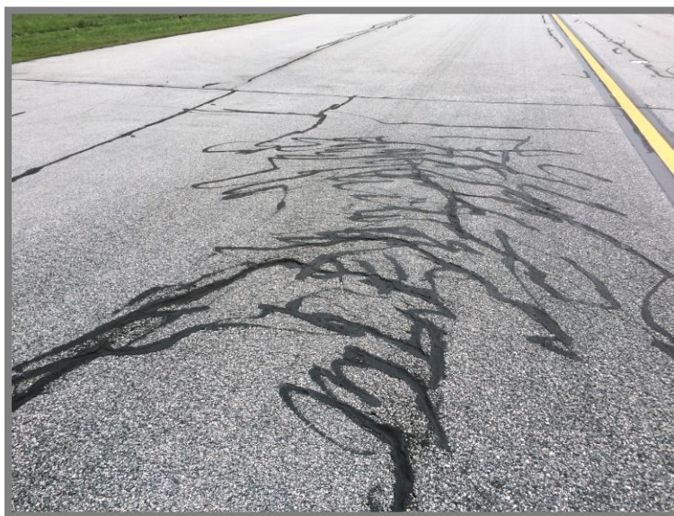
Slippage Cracking – Taxiway G
