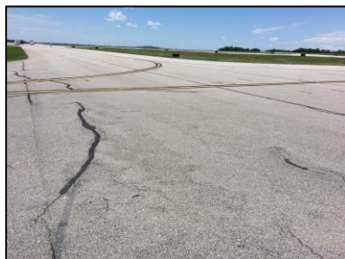
L&T Crack and Swelling
