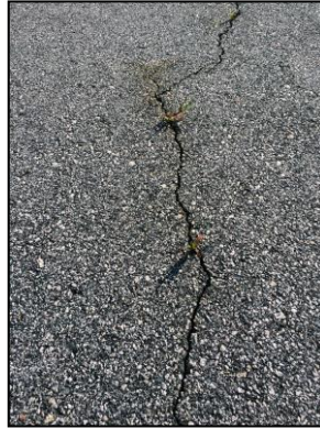
L&T Crack and Swelling
