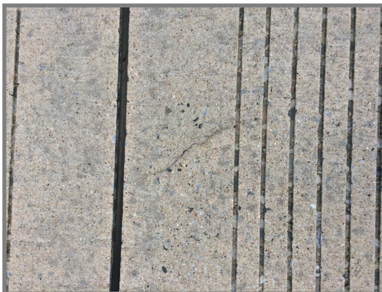
Shrinkage Cracking – Runway 4-22
