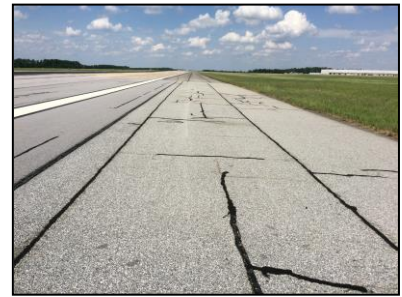
Block Crack and L&T Crack
