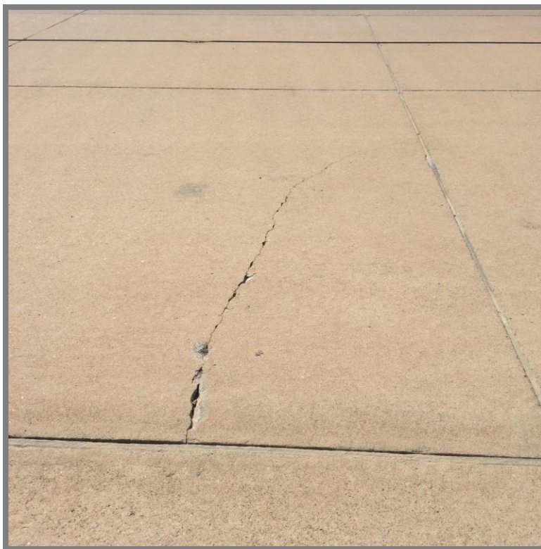
Longitudinal/Transverse/Diagonal Crack – Fire Station Apron
