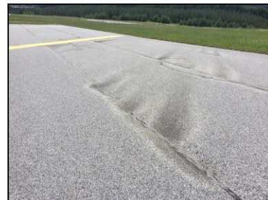
L&T Crack and Swelling
