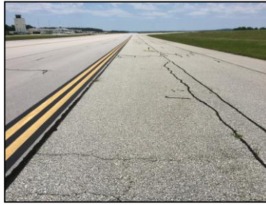
Block Crack, L&T Crack and Swelling
