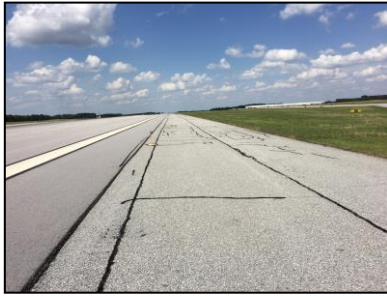
L&T Crack
