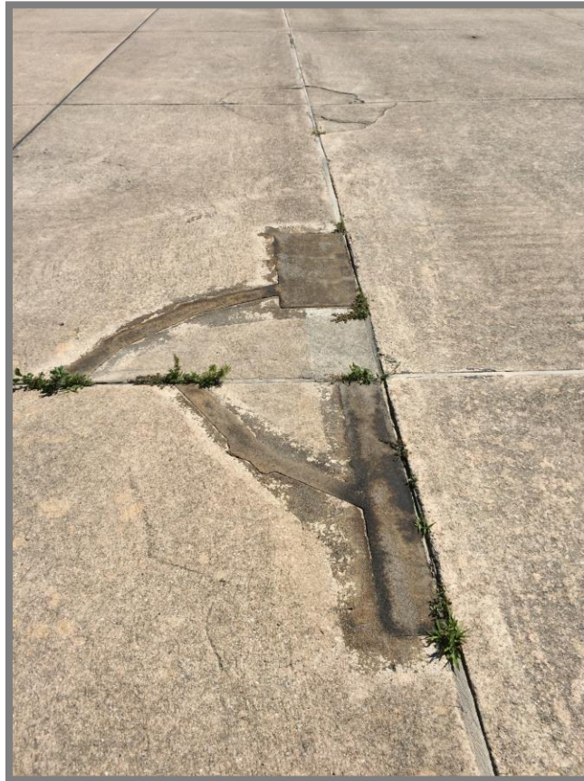
Joint Seal Damage & Patching – Fire Station Apron
