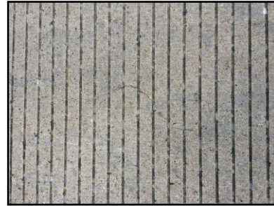
Shrinkage Crack
