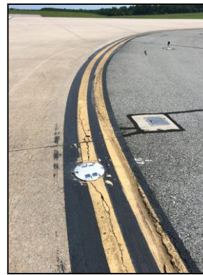
Linear Crack
