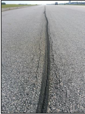
L&T Crack
