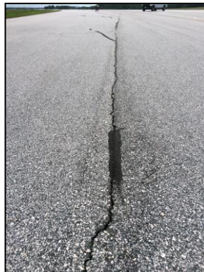
L&T Crack, Weathering, Swelling and Rutting
