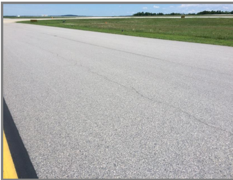
Longitudinal/Transverse Cracking – Taxiway 1
