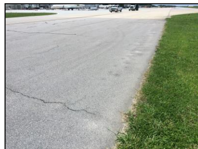
L&T Crack and Swelling
