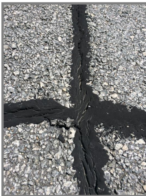
Weathering and L&T Cracking –Runway 4-22 Shoulder
