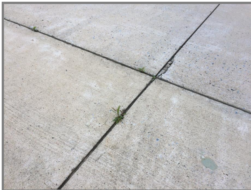
Joint Seal Damage – North Cargo Area
