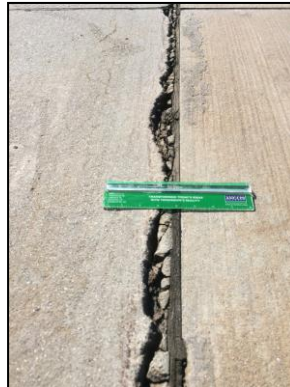
Joint Spall
