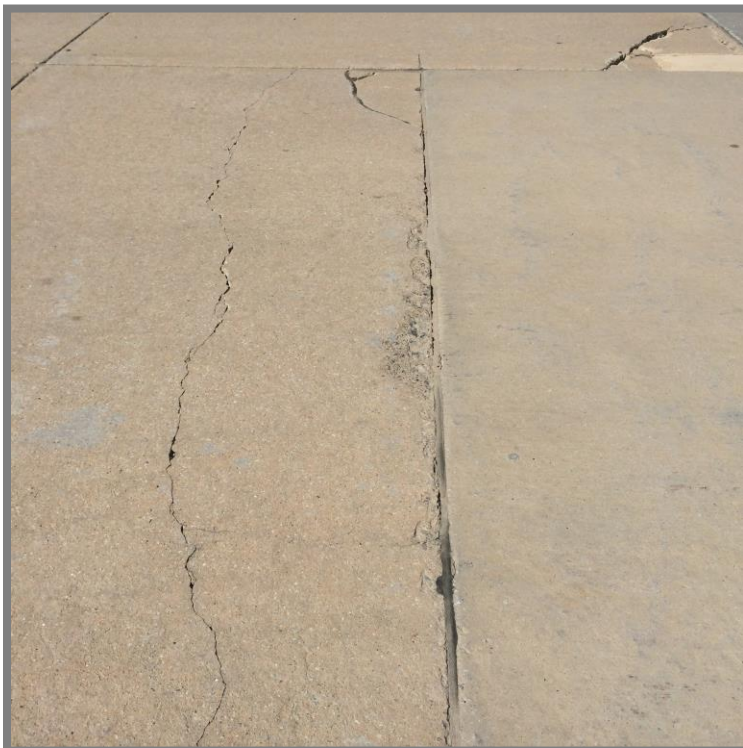
Longitudinal/Transverse/Diagonal Crack – Fire Station Apron
