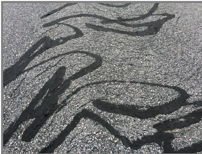
Slippage Cracking – Taxiway G
