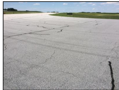
L&T Crack
