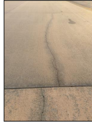
Linear Crack
