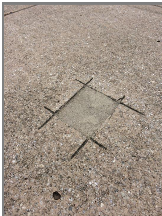
Patching – Air Carrier Terminal Apron
