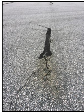
L&T Crack, Weathering and Swelling
