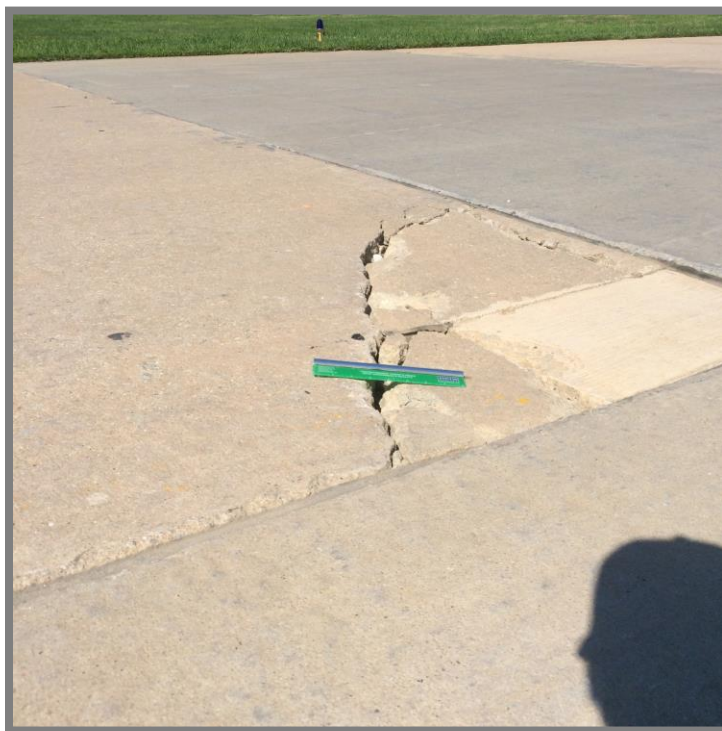
Corner Break – Fire Station Apron
