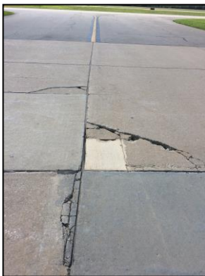
Corner Break and Small Patch
