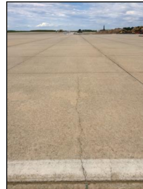
Linear Crack
