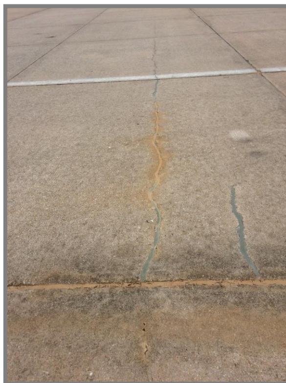
Longitudinal/Transverse/Diagonal Crack – Hangar 1
