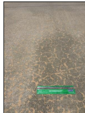
Shrinkage Crack
