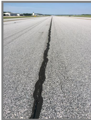
Longitudinal/Transverse Cracking – Taxiway L
