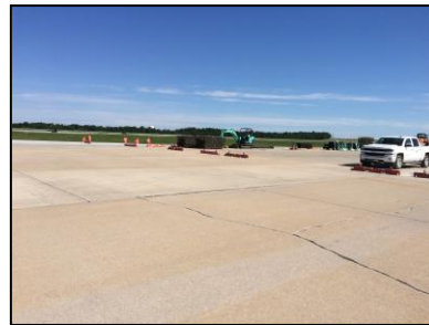
Linear Crack
